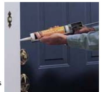
Caulk around the doorway to keep out drafts.
